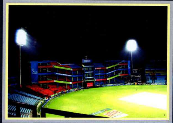
FIROJ SHAH KOTLA CRICKET STADIUM ( DELHI )
