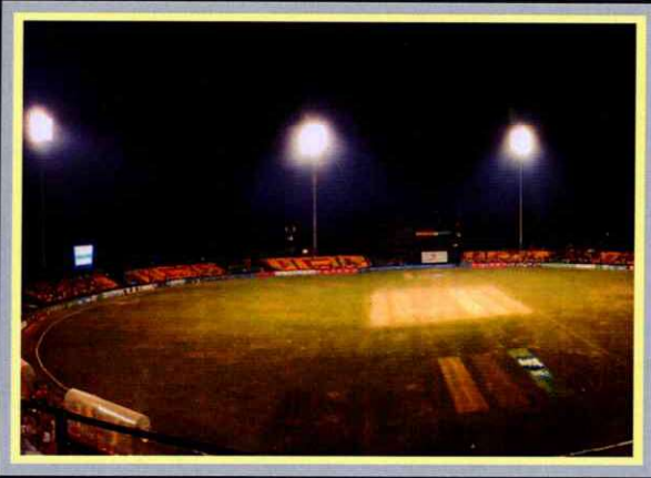
PANCHKULA CRICKET STADIUM (CHANDIGARH)
